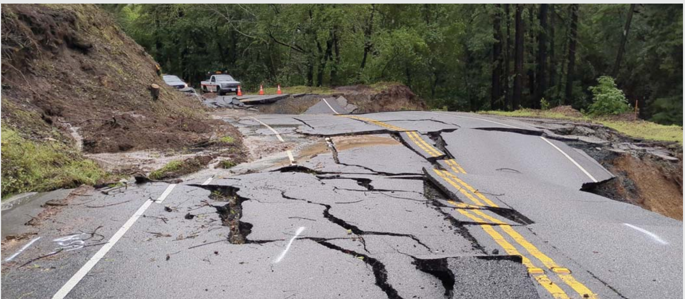
The road to the home zendo
